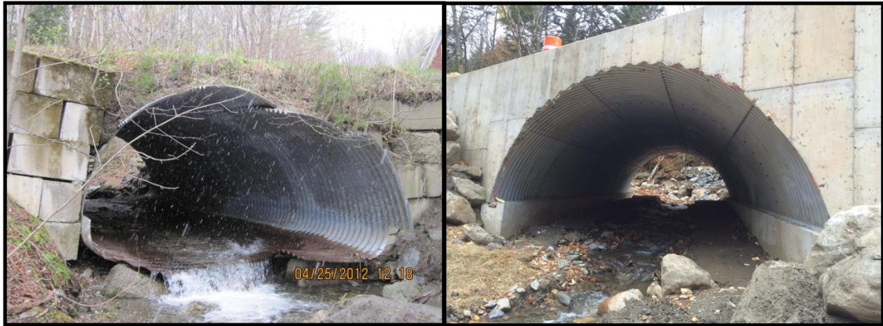
Figure 5. Pre and post culvert replacement photos from Bradley Brook in Warren, VT. Project partners include the Friends of the Mad River, USFWS, USFS, Town of Warren, Winooski Natural Resource Conservation District and VFWD.
