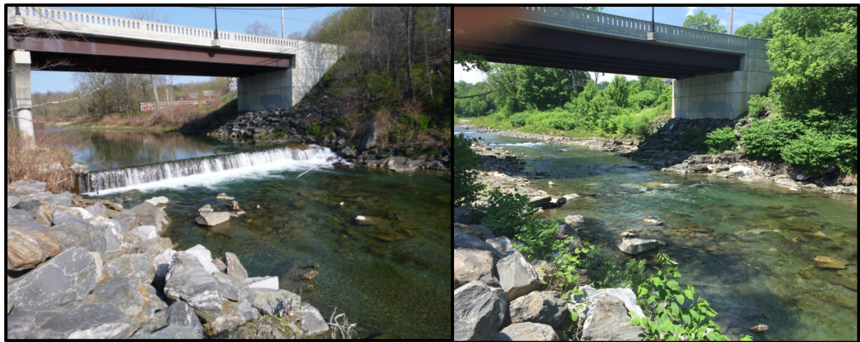
Figure 6. Pre and post photos of the Sargeant Osgood Roundy Dam removal in Randolph, VT. Project partners include American Rivers, TNC, White River Partnership, VDEC and VFWD.
