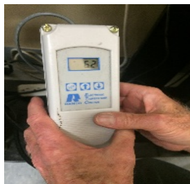
Control unit for chiller
